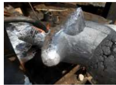
Figure 13.3 welding pieces and filling holes
